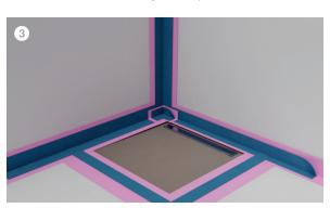
Measure and cut the waterproof tape to size. Apply the tapes, corners and other parts made of sealing membrane. The tape should be applied first, then corners. Tanking liquid can be used as adhesive for them.
