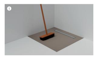
Once the drain is installed and you are ready to proceed to waterproofing, prepare the working area. Remove garbage and make sure you have sufficient space for comfortable work. Clean the floor and walls from dust and debris. Prepare materials and tools necessary to complete the work.
