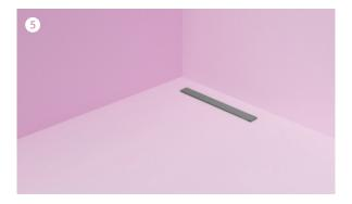
The second coat should cover the same area that the first layer was applied to. Allow the second layer to dry, which should take about 1-2 hours, before proceeding to the next step.
