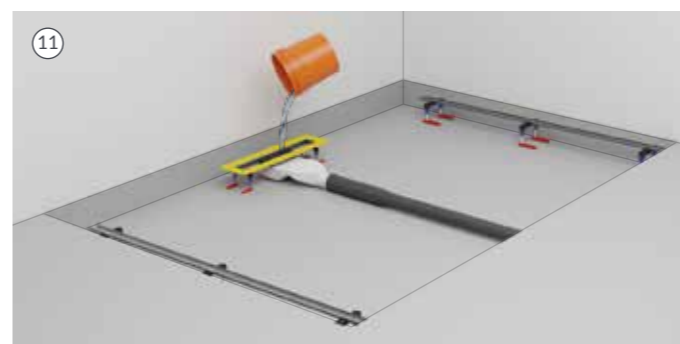
11. Plumb the shower drain to the drainage system and test for leaks.
