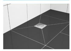
7. Once the liquid foil is completely dry as per the manufacturer's instructions, the shower surface can be tiled (e.g. ceramic tiles or granite). Seal the gap between the tiles and the gulley frame with flexible sanitary silicone compatible with the tile and grout colour.
