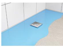
4. Cover the flange and the surrouding area with an insulating foil in a liquid form.
