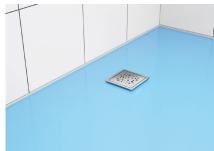
Apply a second coat of the liquid foil to whole surface of the shower area and sealing membrane.
